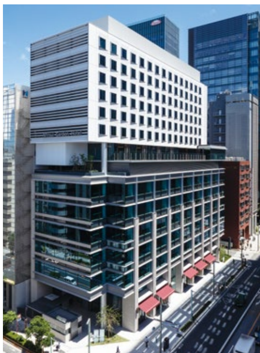
OVOL Nihonbashi Building
