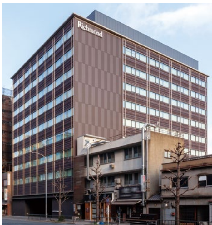
OVOL Kyoto Ekimae Building
