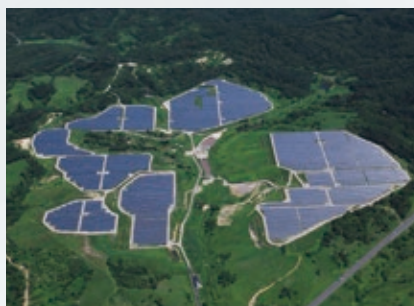
Eco Power JP Co., Ltd. established, marking the group's entry in the renewable energy business. (Kushiro Onbetsu Solar Power Generation Plant)
