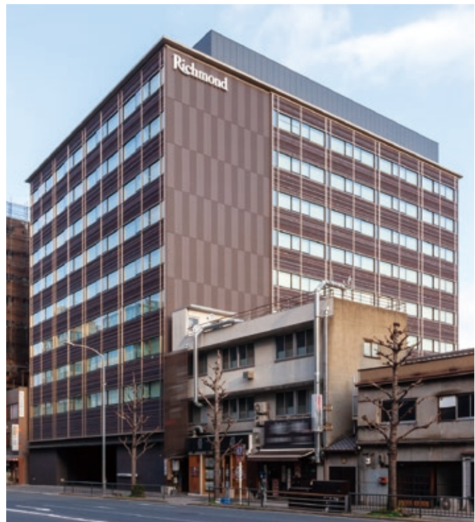
OVOL Kyoto Ekimae Building
