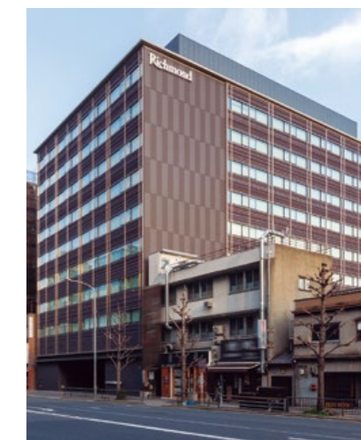
OVOL Kyoto Ekimae Building
