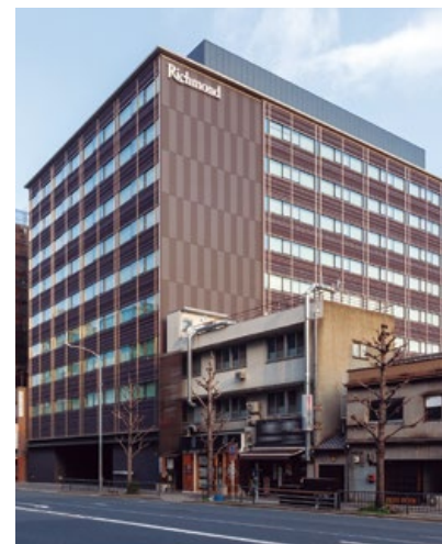
OVOL Kyoto Ekimae Building
