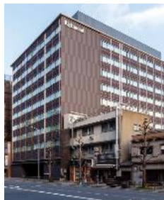
OVOL Kyoto Ekimae Building
