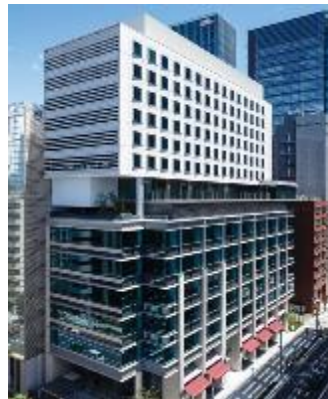
OVOL Nihonbashi Building
