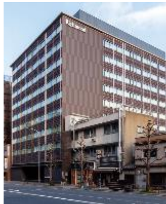
OVOL Kyoto Ekimae Building
