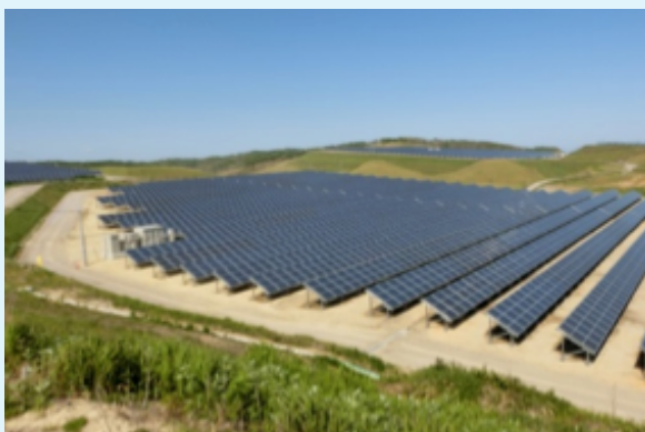
The solar-power generation plant built on an expansive hillside in Kushiro City, Hokkaido
