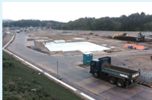
Construction is progressing on a wood-based biomass power plant in Noda Village, Iwate prefecture (Photograph: May 2015)
