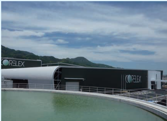
Exterior view of the new mill (Photograph: May 2015)
