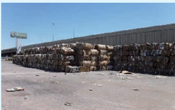
Phoenix Plant of JRS Resources
